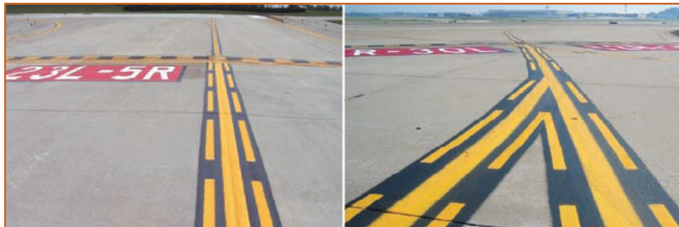
Diagram A: On light pavement, the new taxiway centerline design features reflective glass beads and a solid yellow line outlined in black. The new design is easier for pilots to see in various light and weather conditions.
