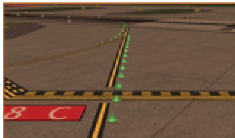
Diagram B: Previously, taxiway centerline lights extended from the apron to the runway with no distinction from lead-on lights. Now, they include alternating yellow and green lights beyond the hold-short line to indicate a runway.
