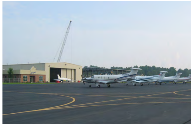
Aircraft on the UZA ramp during construction of a storage hangar.
